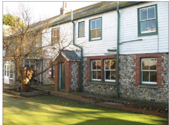
Curtilage listed terraced cottages
